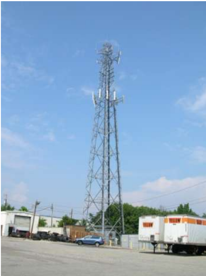
Self-Supporting Lattice Tower
